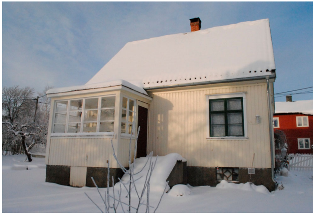
Figure 1. Villa Dammen, Moss, was with its steep saddle pitched roof and classical proportions constructed in a slightly obsolete style. The glass veranda is not heated. Photo: Fredrik Berg.
